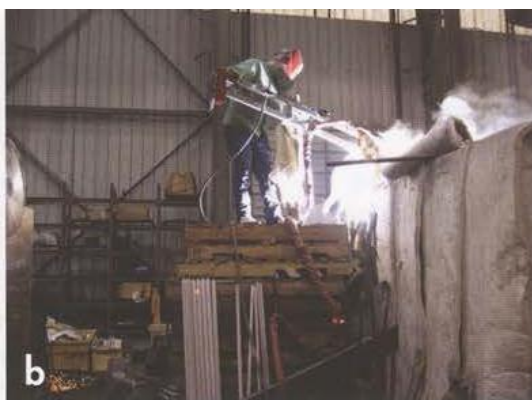
Figure 2 Work man repairs hammer base by welding
