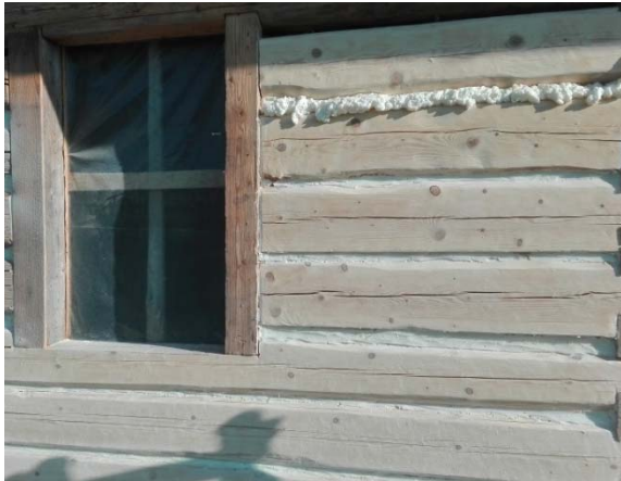
Figure 3. Wall of the house during grinding
