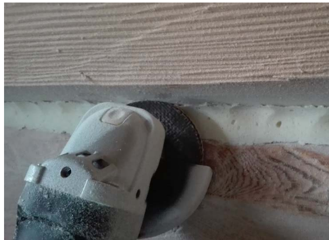
Figure 2. Grinding of the joints
