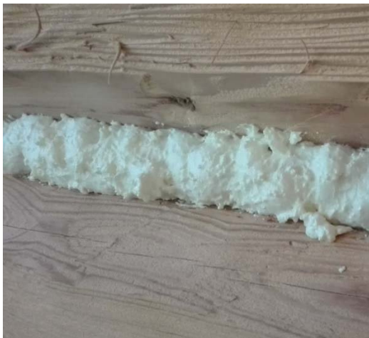
Figure 1. Filling the gaps with a low-pressure sealant
