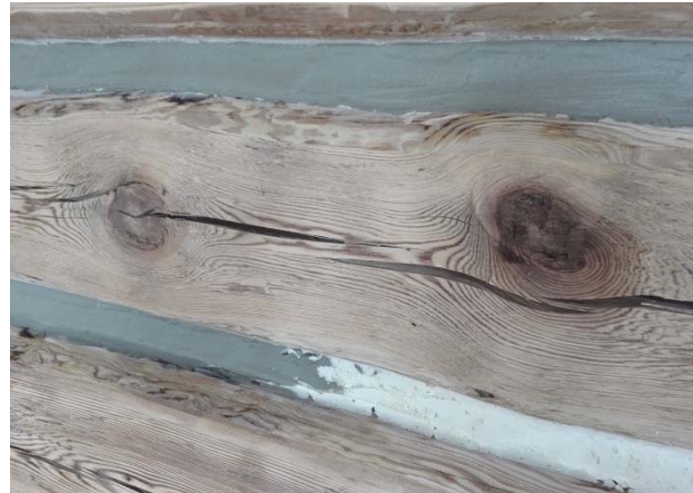
Figure 4. Joints during the application of the adhesive
