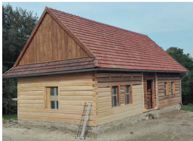
Figure 6. Finished walls with the sealing process completed
